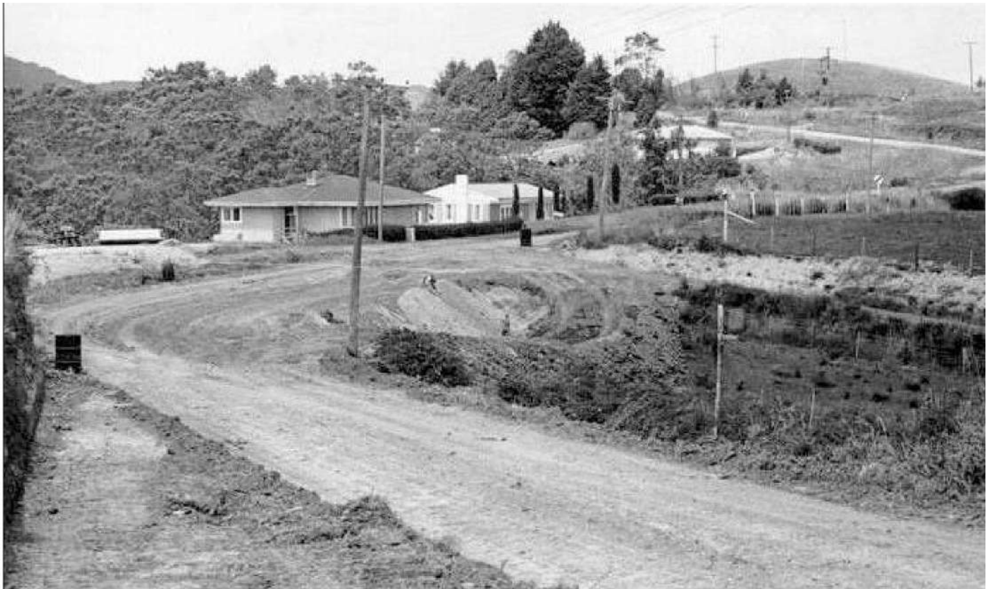
The Kimihia Road correction with the earth movement nearly completed and awaiting metal. The Yates farm is at the top right of the photo. At some time in the future a concrete water supply reservoir was placed on the hill in the distance to supply the increase in residential buildings. The road was originally constructed to service the underground mine in the early 1900s and later the farms that were developed by some of the miners.
