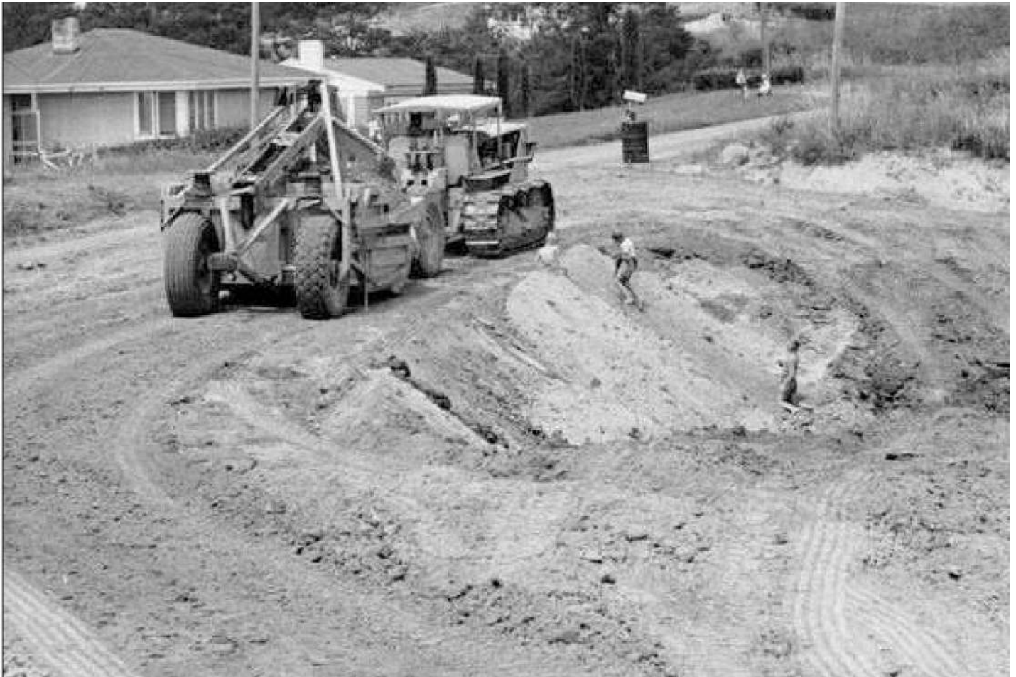
An awkward dip and curve in Kimihia Road, 400 yards east of the Russell Road intersection, being straightened out with heavy machinery from Downer & Company, who also had the contract for running Kimihia opencast mine. The road correction was to facilitate easier travel by the trucks carrying coal from the mine, eliminating a particularly nasty small hill.
