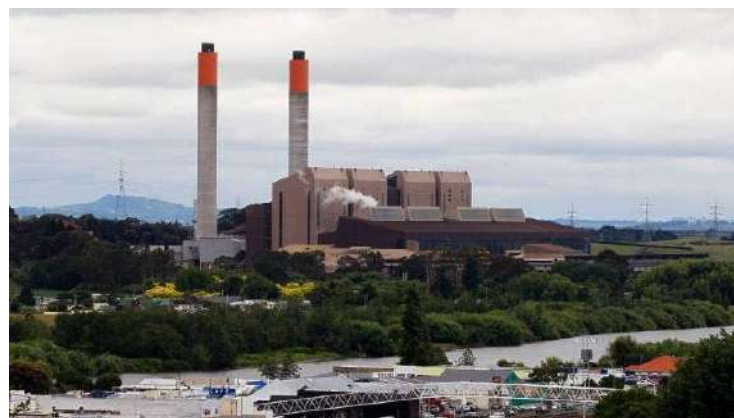
Huntly Power Station..
