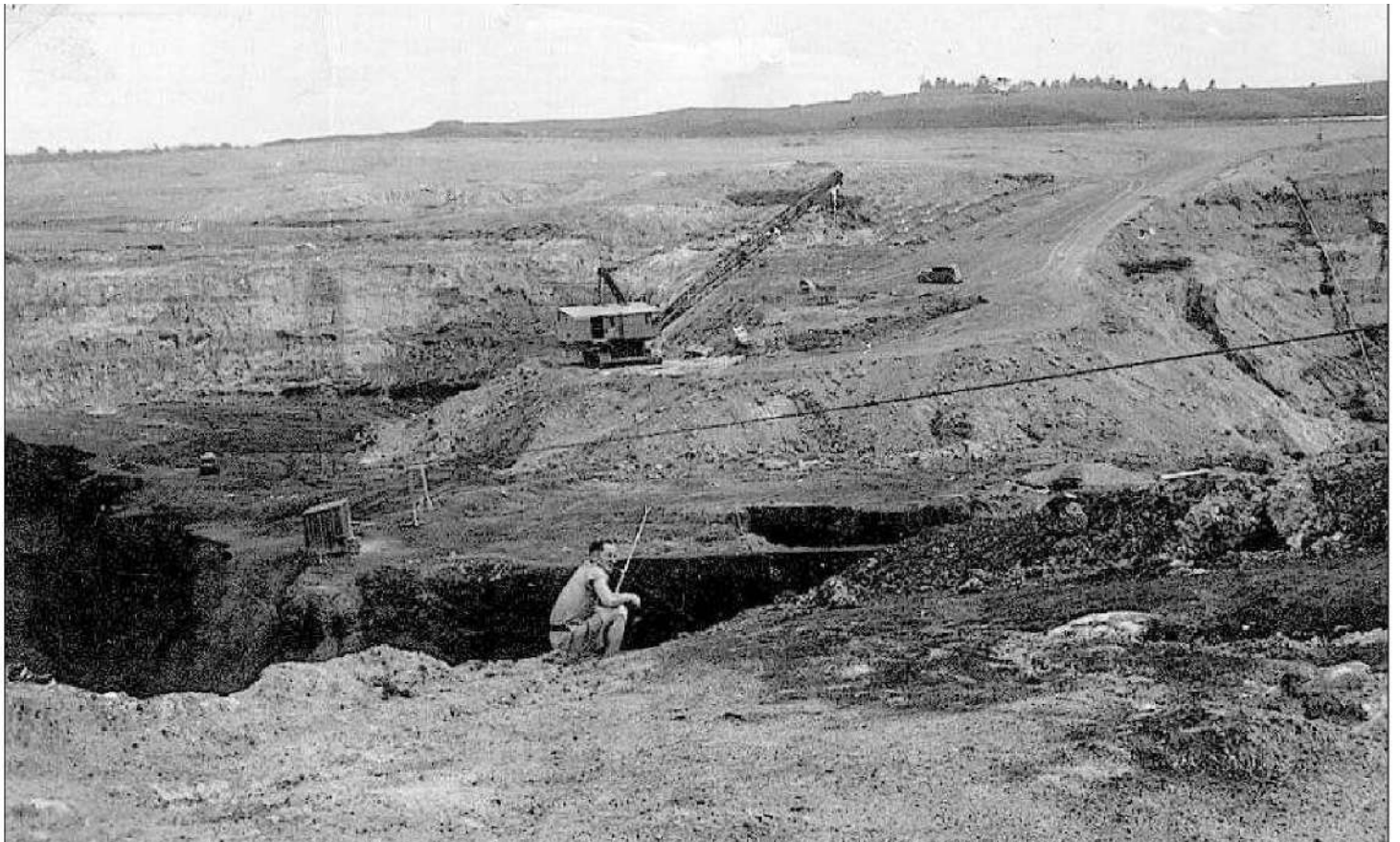
With the 12-B removing overburden in the background, the Flying Fox continued to operate. The steel hawser can be seen running across the picture above the workman. The volume of earth that needed removal can be seen here - all of which was dumped into the existing Kimihia Lake over the coffer dam in the background.
