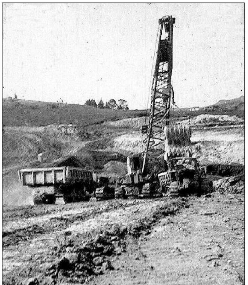
Tractor-pulled Athey wagons line up for overburden removal.
