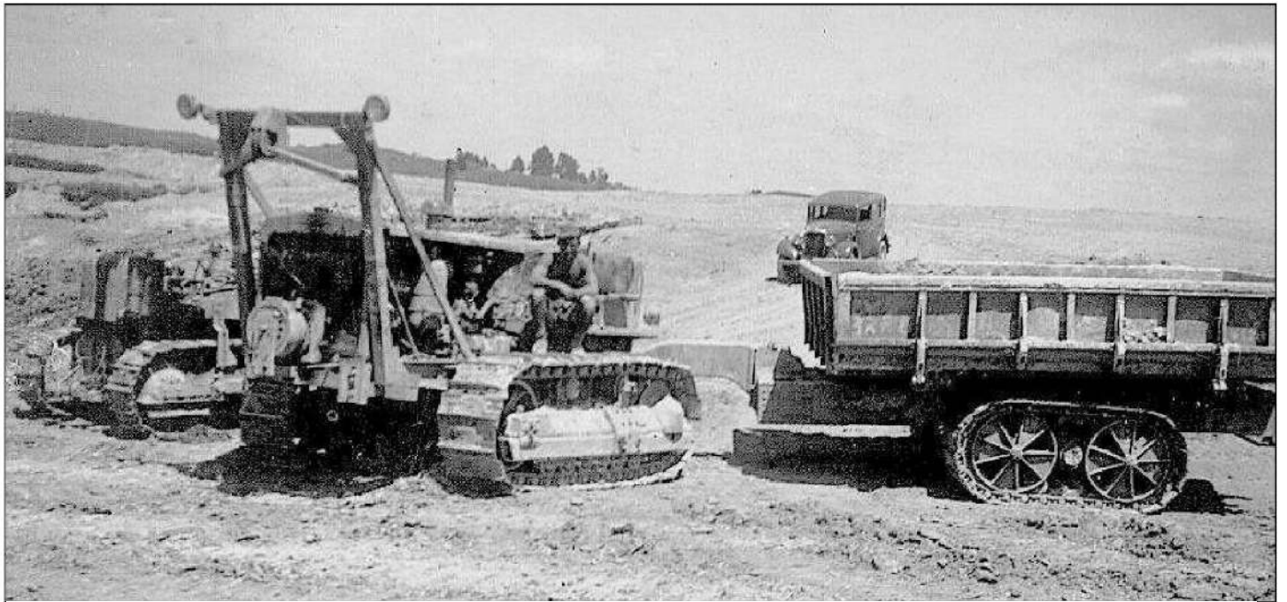
The Athey wagons were used until the very early 1950s, until they were replaced by self-loading carry-alls shown at the bottom of the page.
