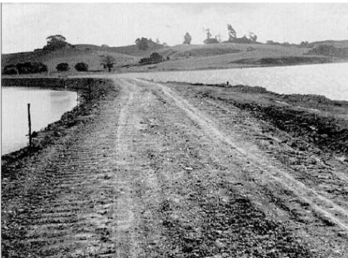
Establishing the major coffer dam for the new pit.
