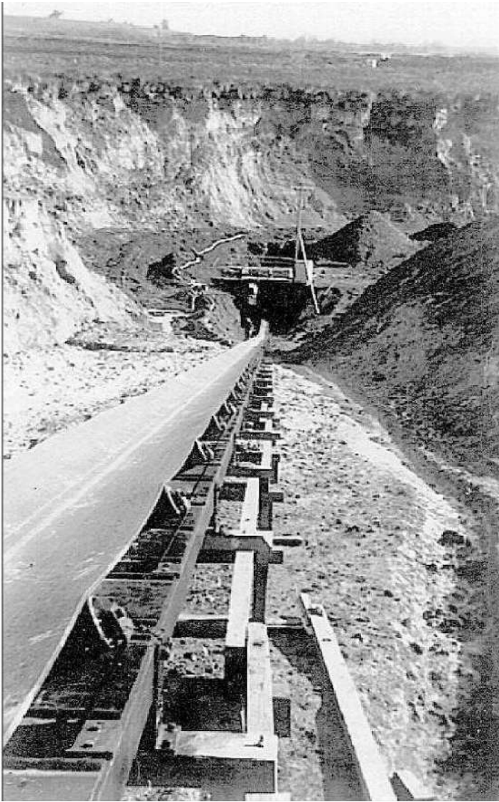
Coal from the pit was transported to the railhead by a rubber conveyor belt.
